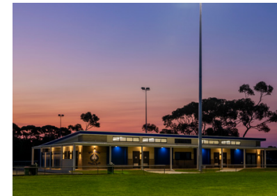
ACHIEVEMENT: Delivering new female friendly change facilities at the Bell Park Sports Club following a $1.95 million upgrade jointly funded by the City and state government. The upgrade also delivered change facilities for officials, a first aid room and storage spaces.
