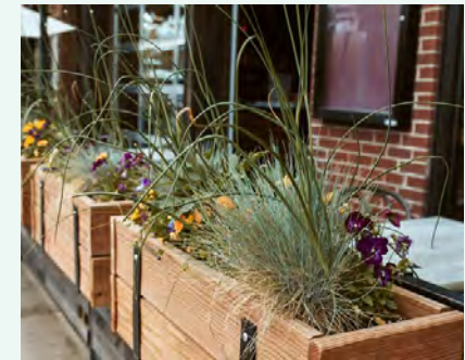
Image 09. Example of planters integrated with barriers with allowance for drainage and clearance for footpath maintenance.
