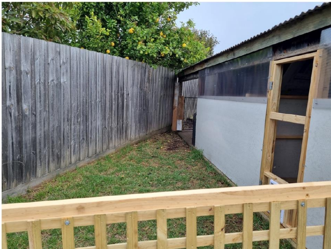
Figure 5 – View along eastern boundary / Eastern elevation of existing garage
