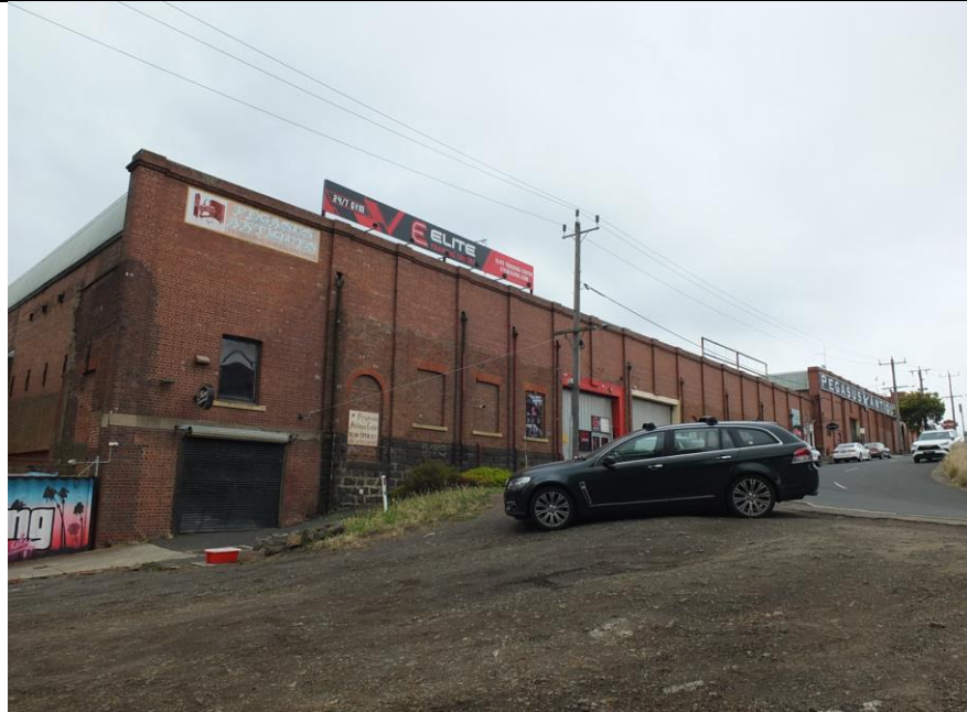
Former Albion Mill, east and part south elevations, December 2023. Source: David Rowe.
