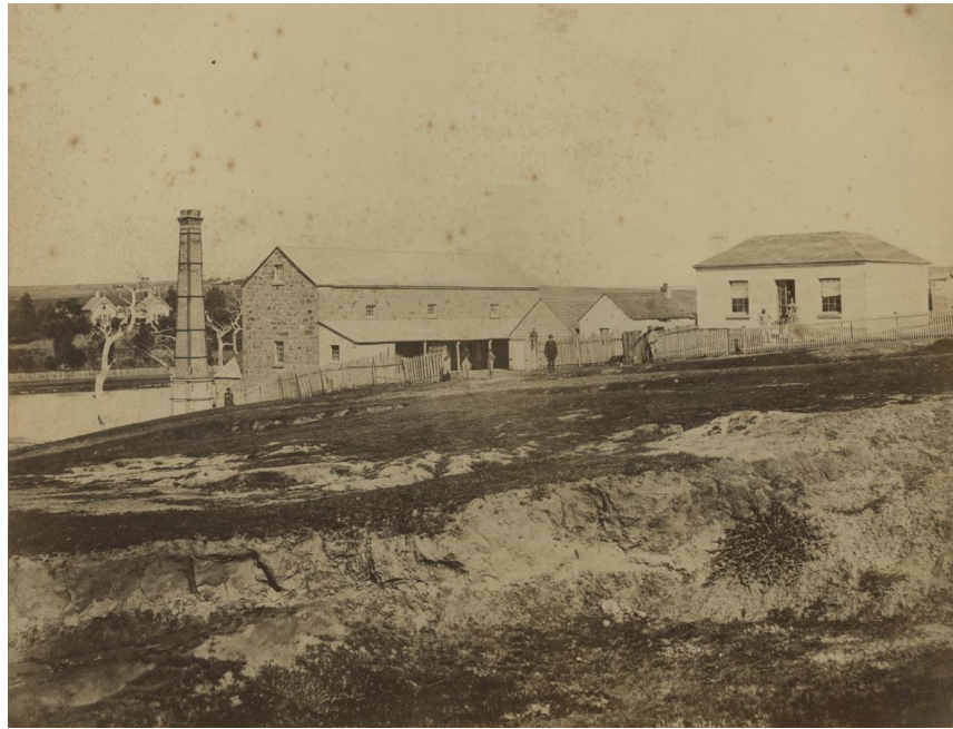
J. Norton, Gray's Flour Mill, Geelong, c.1866. Source: GRS 2009/02172, Geelong Heritage Centre Collection.
