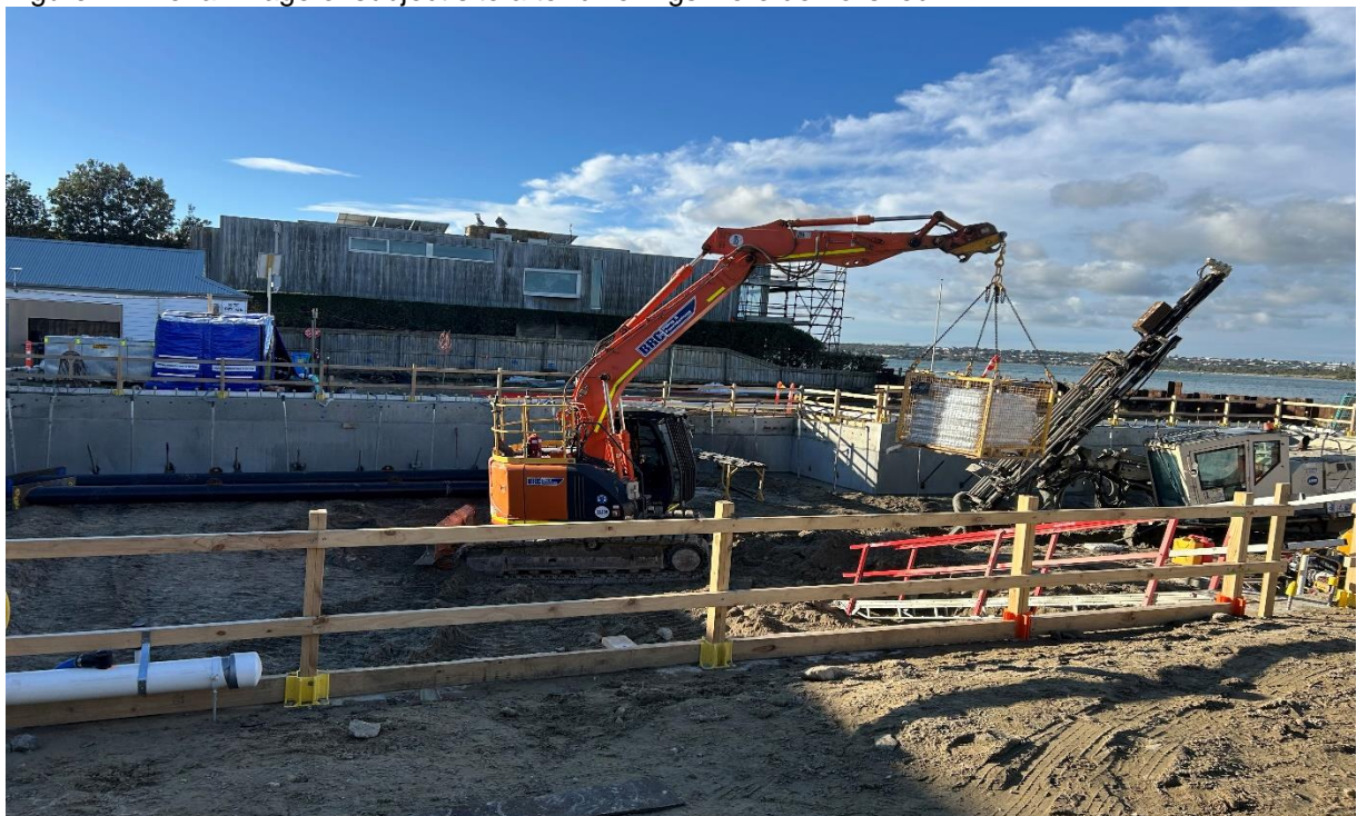
Figure 5 – Subject site showing construction works being carried out.
