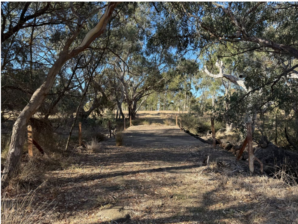
Figure 2. Direct view of the Ripley Weir looking north from the southern embankment. Source: City of Greater Geelong, February 2025.
