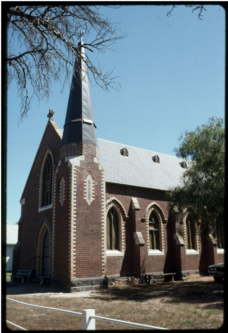
Figure 6. St. Paul's Lutheran Church in 1976. Source: State Library of Victoria, Collins, J. T. (1976). St. Paul's Lutheran Church, Torquay Road, Grovedale.
