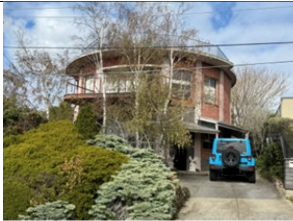
View of the building's façade. Source: City of Greater Geelong, May 2025.
