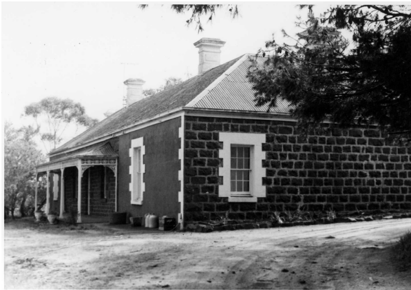
Figure 3. Oblique view of the façade and eastern side elevation. Source: State Library Victoria, Collins, J. T. (1977). Moorabool Craigton.
