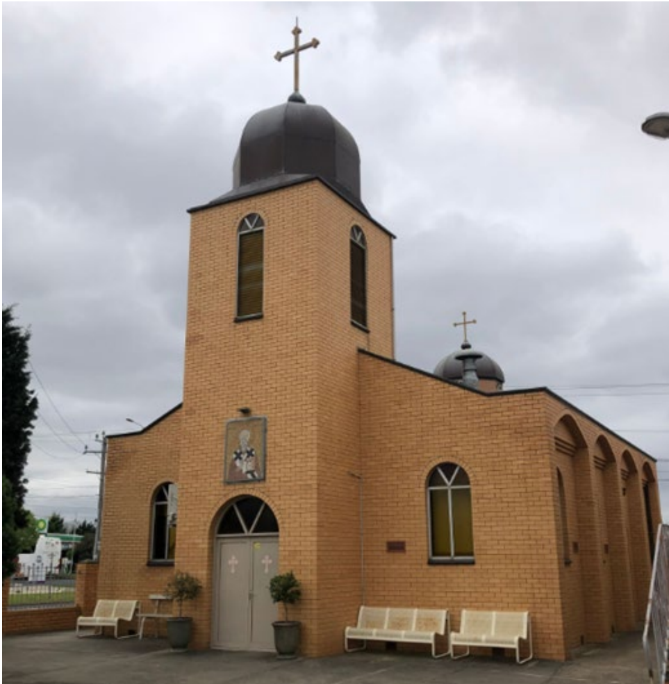
Figure 2. Oblique view of the St Nicholas Serbian Orthodox Church at 124 Ballarat Road, Hamlyn Heights. Source: City of Greater Geelong, September 2024.
