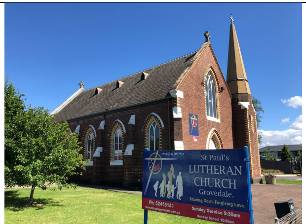
Oblique view of St Paul's Lutheran Church looking northwest. Source: City of Greater Geelong, November 2024.
