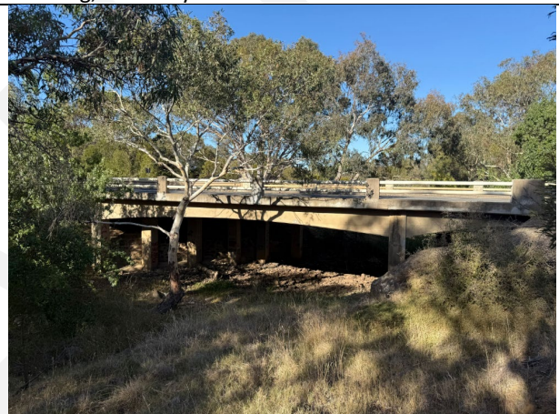
Non-contributory 1928 bridge. Source: City of Greater Geelong, February 2025
