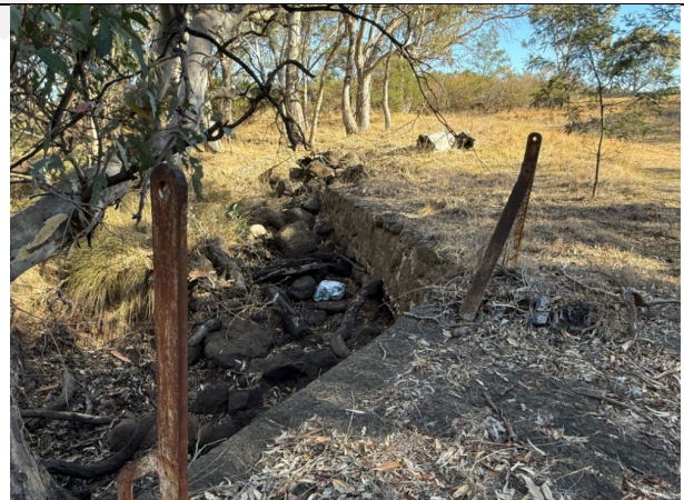
Oblique view of two of the steel boundary posts. Source: City of Greater Geelong, February 2025.
