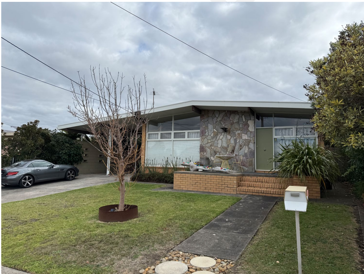
Figure 2. Oblique view of the building's façade, looking northwest. Source: City of Greater Geelong, 2025.
