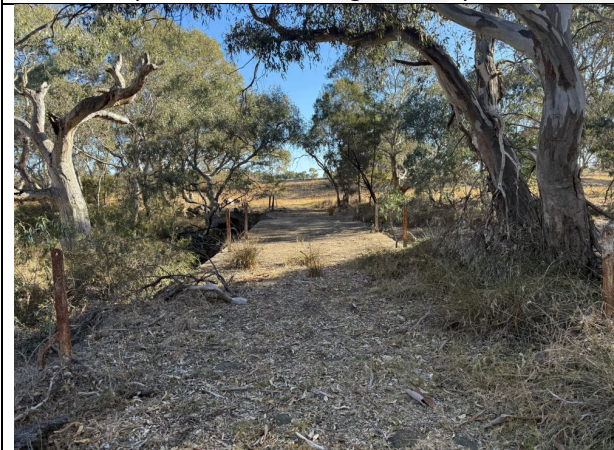
Direct view of the Ripley Weir looking south from the northern embankment. Source: City of Greater Geelong, February 2025.
