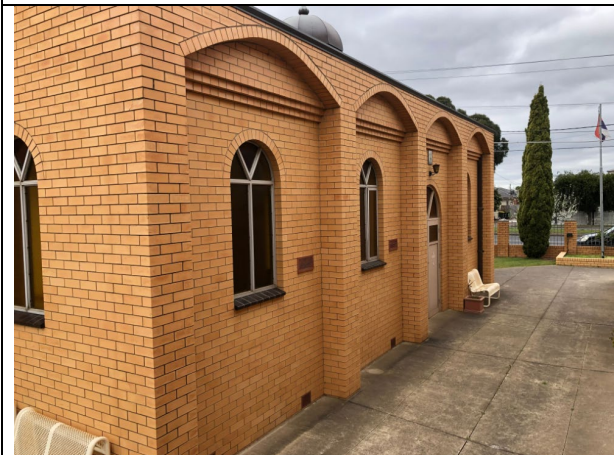
Oblique view of the southern elevation of the church. Source: City of Greater Geelong, September 2024.
