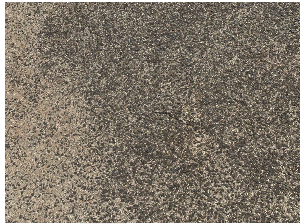
Detail view of the coarse aggregate reinforced cement. Source: City of Greater Geelong, February 2025
