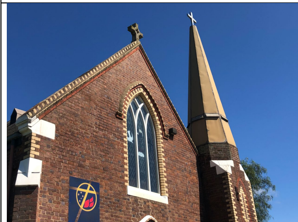
Overview of the facade. Source: City of Greater Geelong, November 2024.
