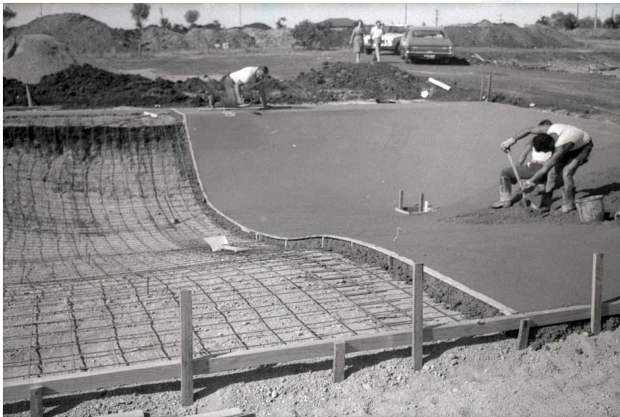
Figure 3. 1980 image showing the construction of the bowls. Source: Geelong Regional Libraries.
