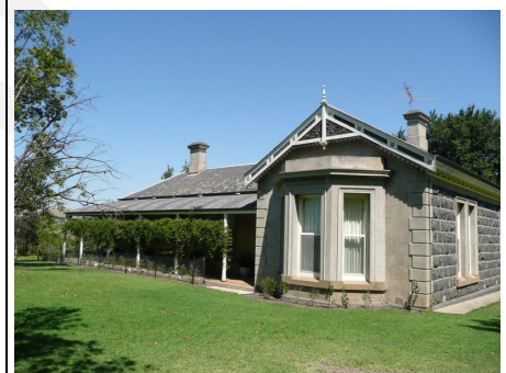
Figure 15. Frogmore, 425-465 Hamilton Highway, Fyansford. Source: Victorian Heritage Database
