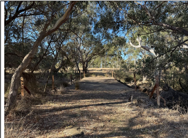
Direct view of the Ripley Weir looking north from the southern embankment. Source: City of Greater Geelong, February 2025.
