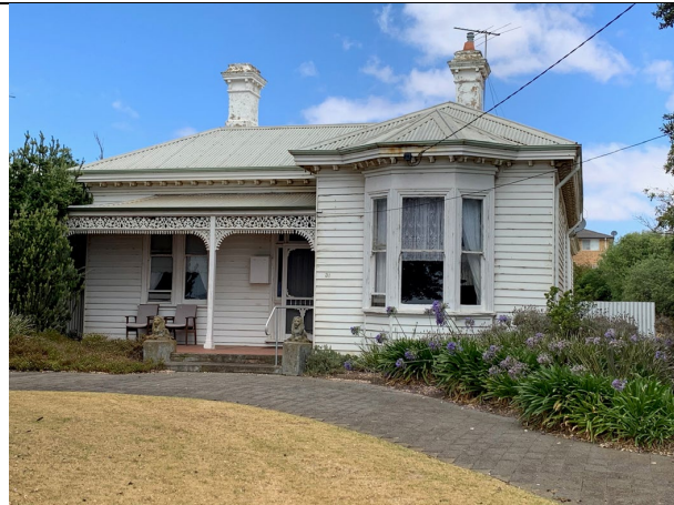
Direct view of Oakrest. Source: City of Greater Geelong, February 2026.
