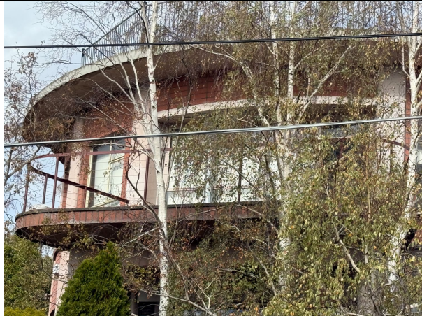
Detail view of the balcony. Source: City of Greater Geelong, May 2025.
