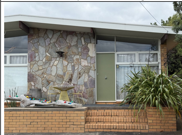
View of porch and entrance looking north. Source: City of Greater Geelong, 2025.
