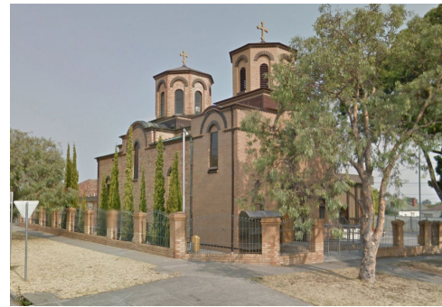
Figure 7. St George Serbian Orthodox Church, 6 Kate Street, St Albans. Source: Google Streetview, April 2023
