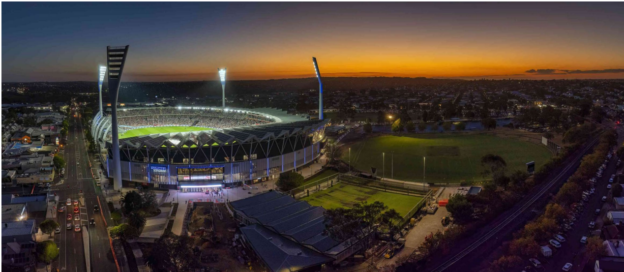
Figure 4. Kardinia Park in South Geelong
