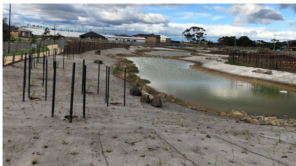
Waurn Ponds constructed waterway – Hams Rd
