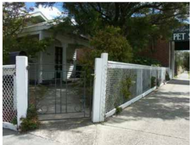
Figure 84 Interwar bungalow styled dwelling with a capped timber post and chain mesh front fence having open geometric steel gate.
