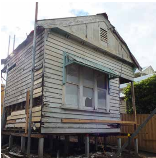
Figure 9 Dwelling, Geelong. Partially retained, restored and repaired dwelling that was safeguarded during demolition and construction.
