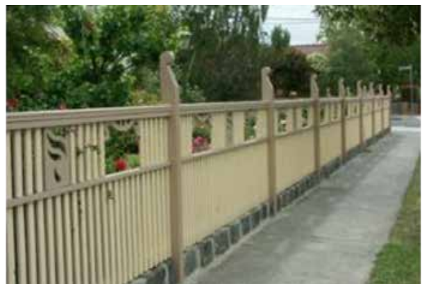
Figure 76 Details of Federation era picket fence with fretwork capping.
