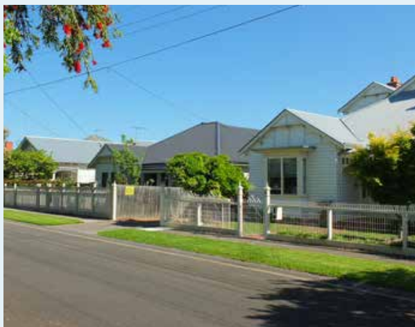
Figure 25 Dwelling, Drumcondra (centre). An example of conservative middle infill.
