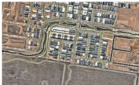
Banksia Estate constructed waterway – Armstrong Creek
