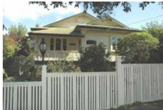
Figure 90 Fence stepped along slope of boundary.
