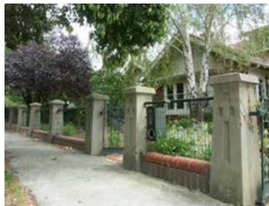
Figure 80 More substantial woven wire fence to large property with rendered piers and brick plinths.
