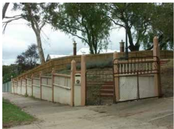
Figure 78 Detail of Federation era ripple iron and timber fretwork fence, with scrolled metal and wire vehicular and pedestrian gates.
