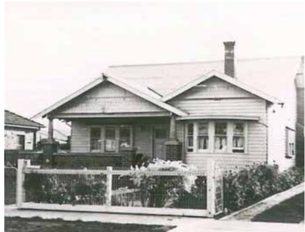
Figure 83 Timber post and rail, and woven wire fence to an interwar bungalow styled dwelling.
