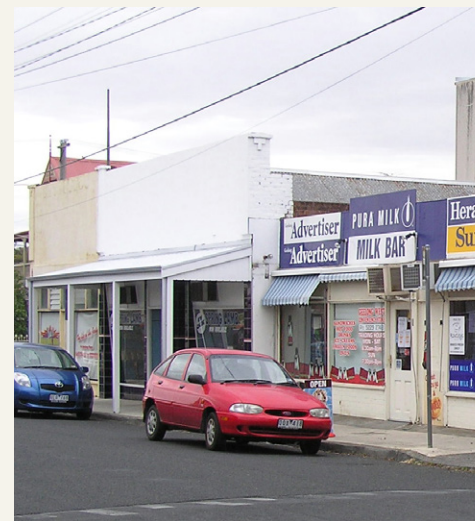
Former Butcher's Shop, 66 Elizabeth Street, Geelong West, 2009
