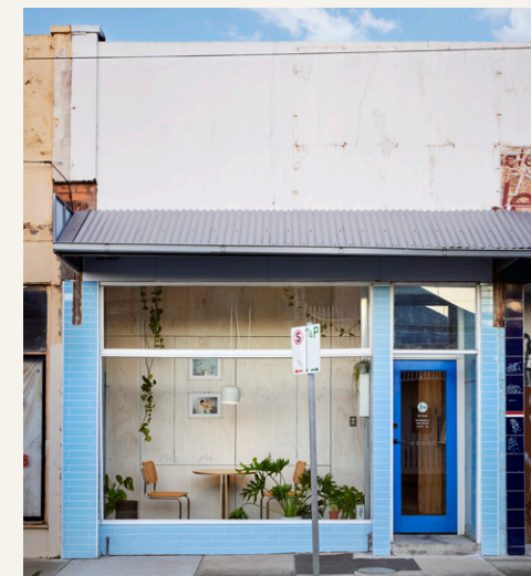
Adapted and restored former shop, 66 Elizabeth Street.
