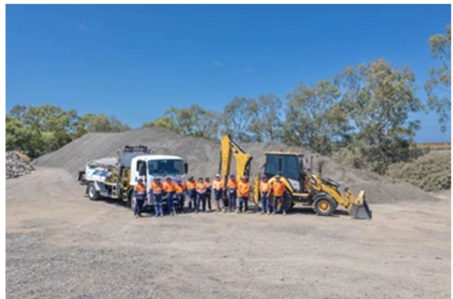
Asphalt after being crushed into road base
