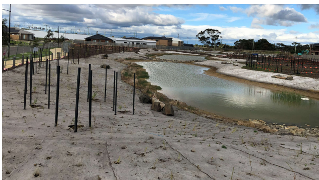
Waurin Ponds constructed waterway – Hams Rd
